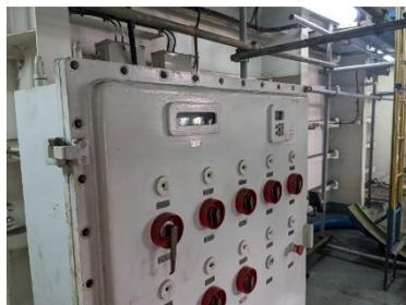
review of lighting, PA/GA speakers and ventilation arrangements. A review of the control panels identified inconsistencies due to equipment modification and incomplete certification. Updating of the rig's hazardous area drawing and hazardous area equipment register was also required.
